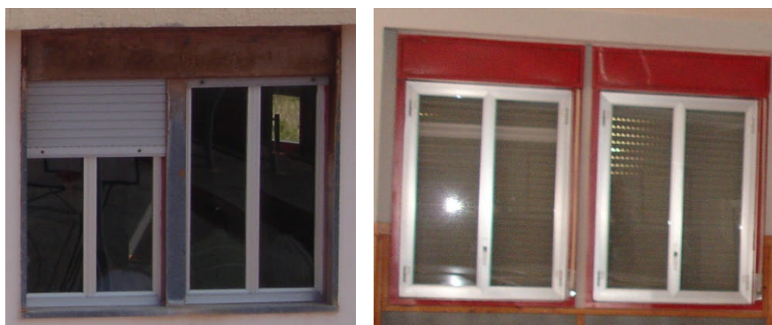
Windows with double door opening
